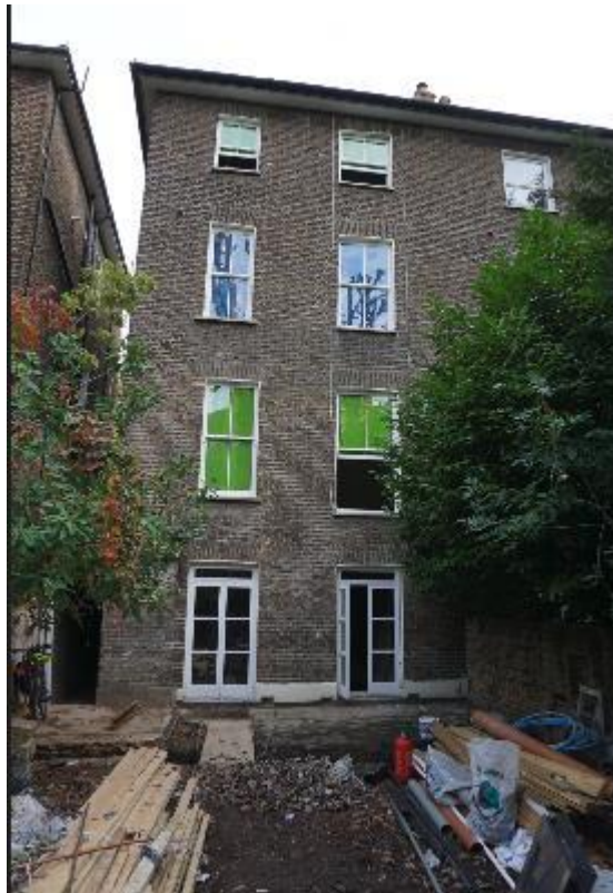
Photo of rear elevation (showing rear shed structure removed)
